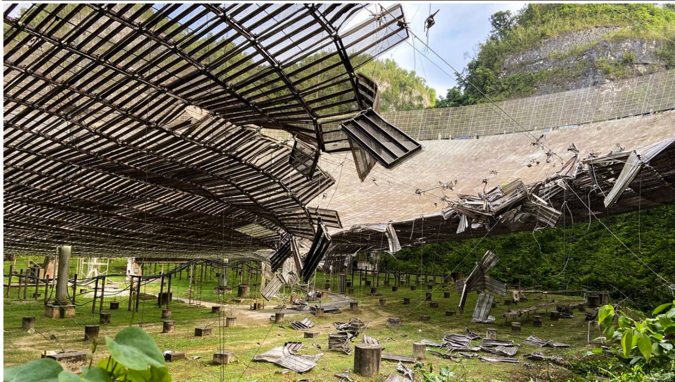
The iconic Arecibo Observatory's giant radio telescope dish suffered serious damage on Aug. 10, 2020 when a support cable broke. (Image credit: University of Central Florida)
