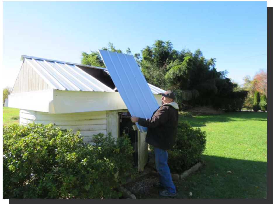
Removing the Panel from the Replacement Peaked Roof
