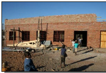
New Community Centre Underway in Bende Mutale
