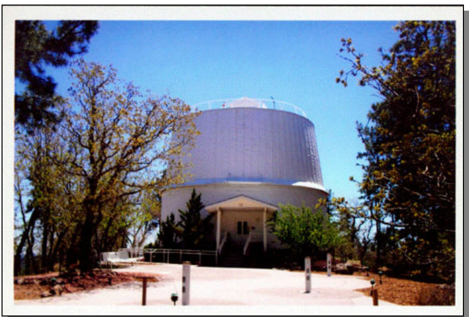
The Lowell Observatory is housed in a 40' building on the outskirts of Flagstaff.
