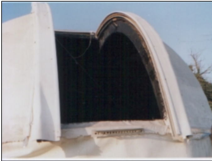
The observing slit in the dome (note the angle bracket at the bottom of the slit that serves as a doorstop for the cover).
