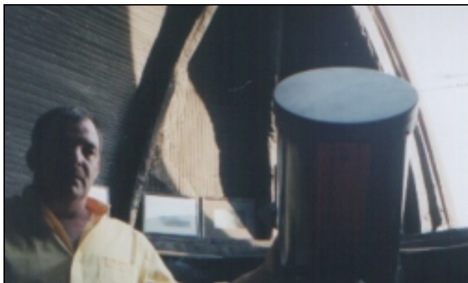
Behind Pete and his beloved Celestron CGE-11, inside the observatory, you can see the R4 insulation (as used on air-conditioning ducts) that Pete used to keep the dome from sweating on the inside. The inside walls were painted flat black to minimize stray light reflections.
