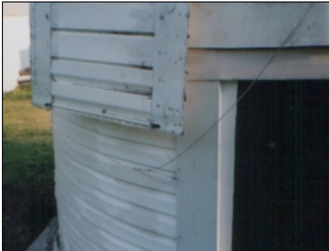
Here you can see the end of the cover for the observing slit hanging down on the other side of the dome, opposite the observing slot. You can also see the light rope used to pull the cover into the "open" position. There is another cord on the other end to pull it closed; the slot cover is not motorized.
