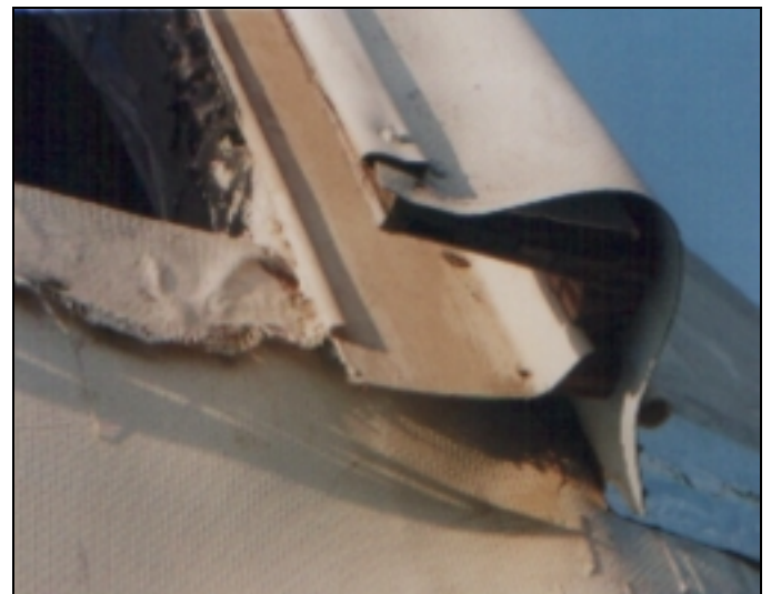
Pete also used some of the swimming pool cover to add a flexible weather strip along the outside of the door guide rails for the dome's observing slot cover door.
