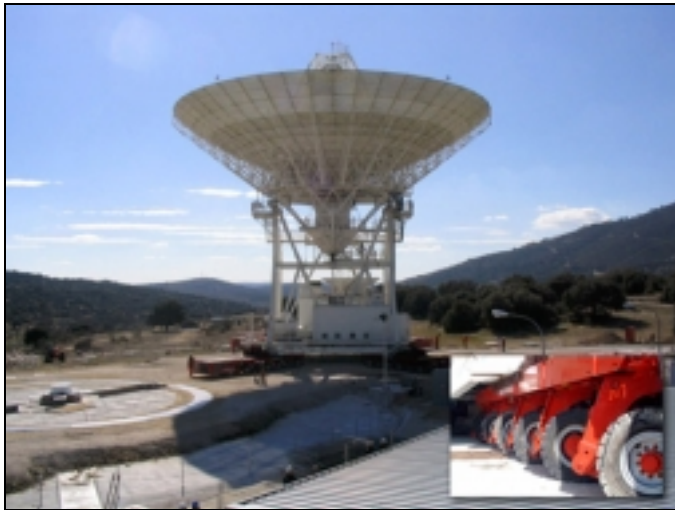
Giant Deep Space Network antenna in Madrid is moved using four 12-axle, 24-wheel crawlers.
