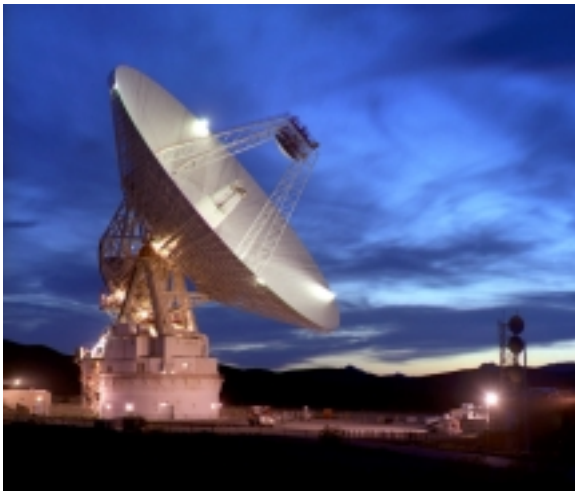
The 70-meter radio "dish" antenna at NASA's Goldstone Station of the Deep Space Network. How big is 70 meters? By comparison, the small rectangular thing near the base, under the front end of the dish, is a maintenance vehicle the size of a pickup truck.
